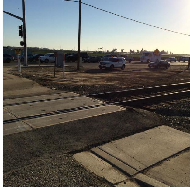
Driver's view to the right, looking at tracks.
